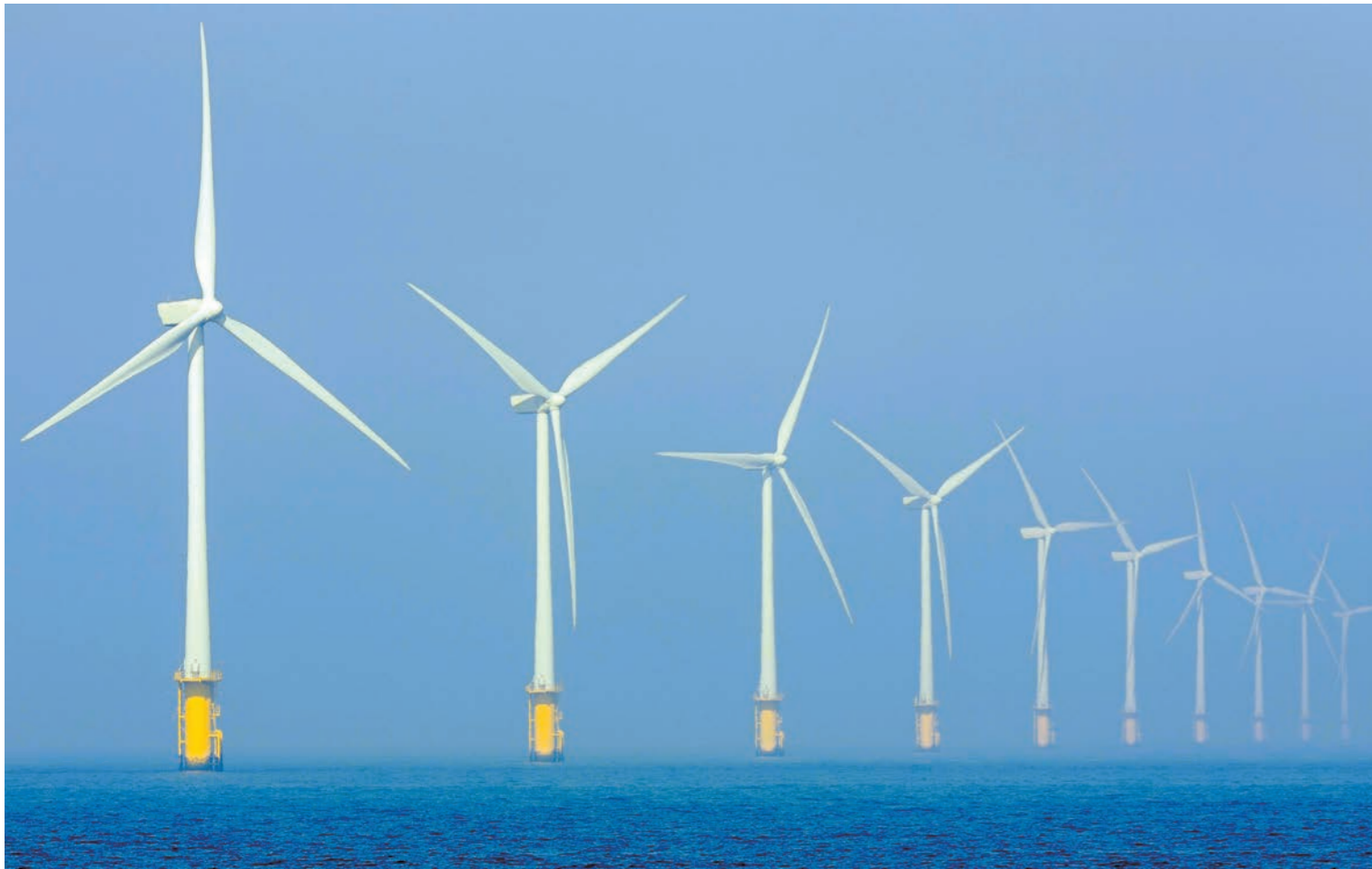
Wind turbines at sea
