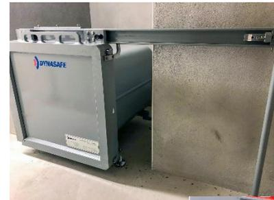
The DynaLOCKR F7 and F10 are designed to serve a wide variety of needs for the explosives engineering, blasting, drilling, mining, fireworks and pyrotechnic industries. They are considered to be urban magazines where small amounts of explosive materials are stored. The DynaLOCKR F7 is a one-drawer explosive storage chamber system that can contain a 2kg TNT equivalent charge. The DynaLOCKR F10 is a two-drawer explosive storage chamber system that can contain a 2kg TNT equivalent charge .
